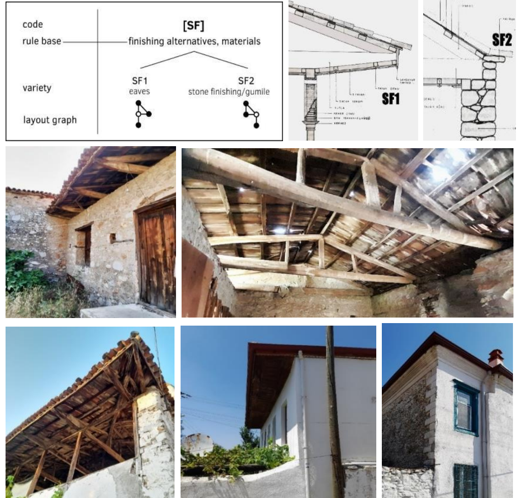
Figure 6. Roof structure and eaves
