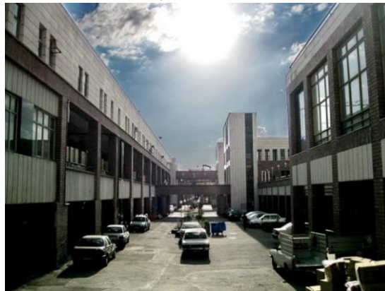
Figure 8. Mashroteh Complex in the Historic Bazaar of Tabriz
