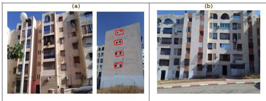
Figure 14. (a) Facade of housing type PRH variant 3 Transformations with creation of openings for sanitary facilities, (b) Facade of housing type PRH to NU8 variant 1, 2 shows the different transformations in facade
