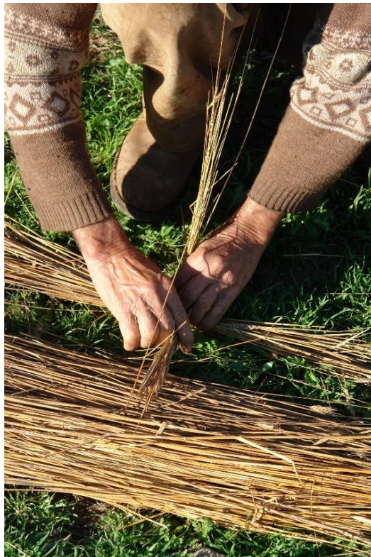
Figure 1. Master preparing a thatched roof. Malhão, Loulé, Algarve
