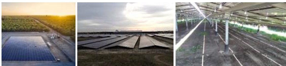
Figures 20, 21, 22. Highest-density ground-mounted PV: flat and wrinkled
