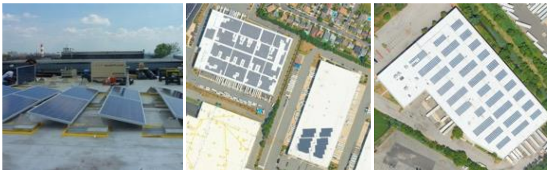
Figures 5, 6, 7. A selection of discontinuous PV arrays on flat roofs
