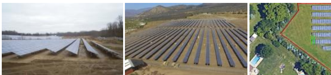
Figures 23, 24. Common topologies of LoCoPV: fixed south-facing; single-axis trackers; Figure 25. diagram comparing array and site power density
