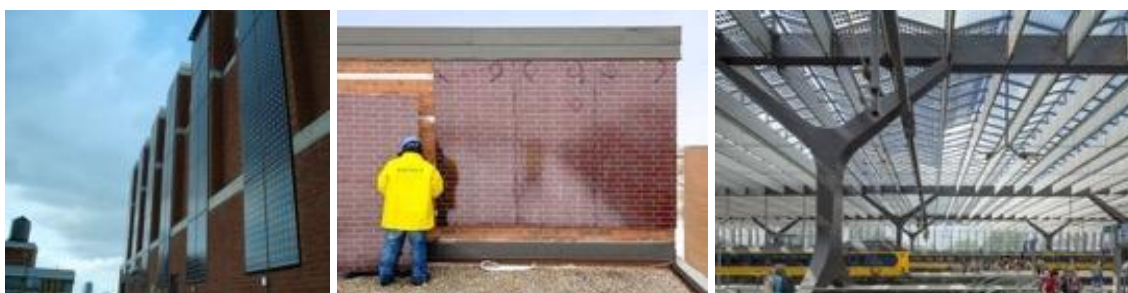
Figure 17. Uncamouflaged BIPV façade with standard modules (2004); 18. brick-mimicking BIPV (2022); 19. semi-translucent BIPV roofing (2014)
