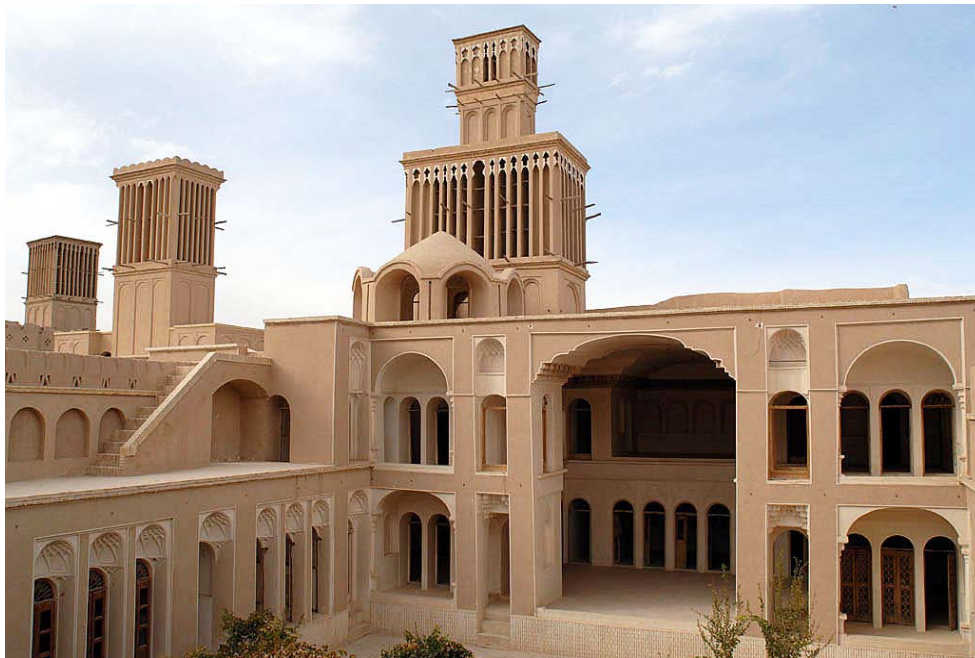
Figure 10. Porch (Eivan) in Aghazadeh House - Abarkooh
