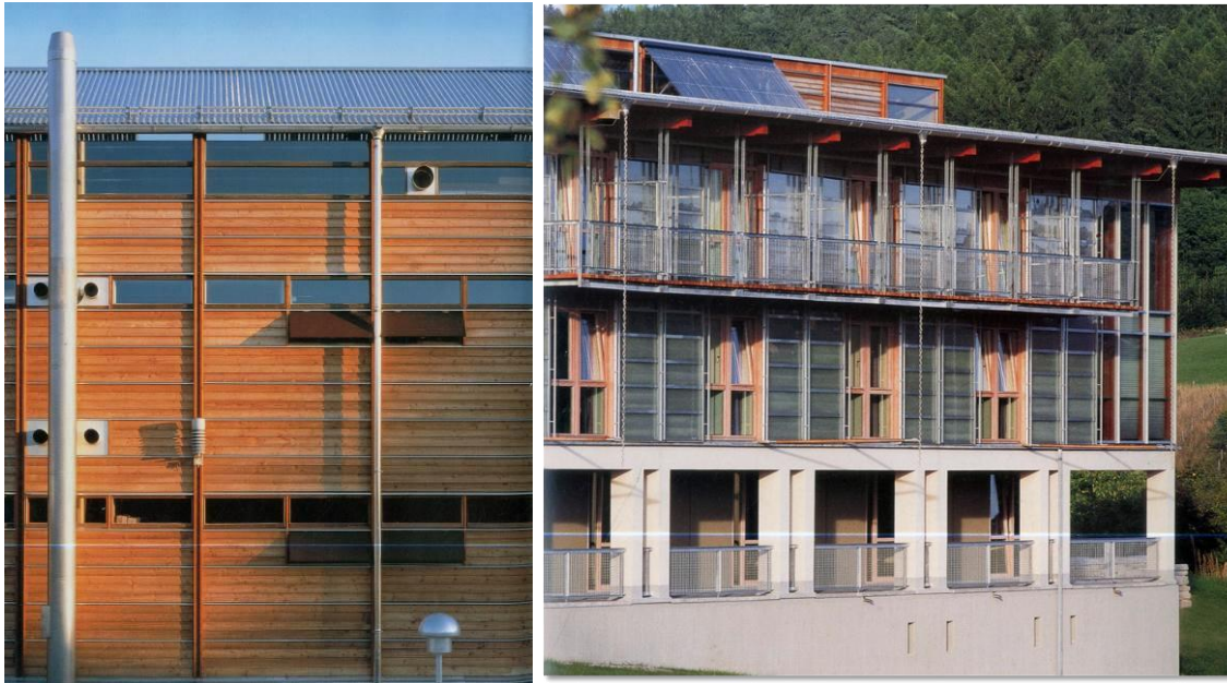
Figure 16. Guest Building, Windberg, from left to right: northern and southern facade
