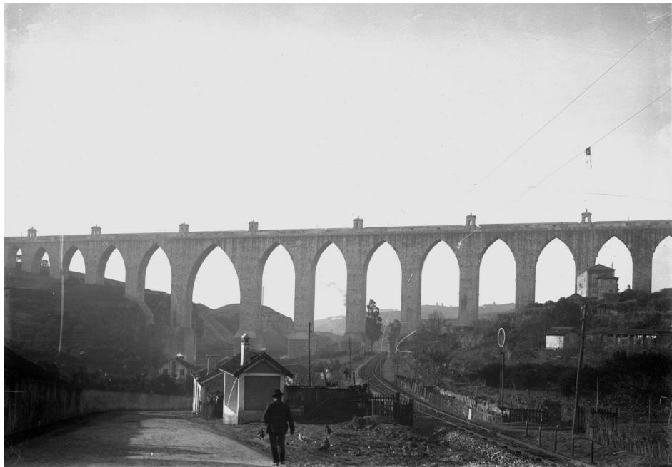
Figure 2. Lisbon Aqueduct in Alcântara valley in 1912
