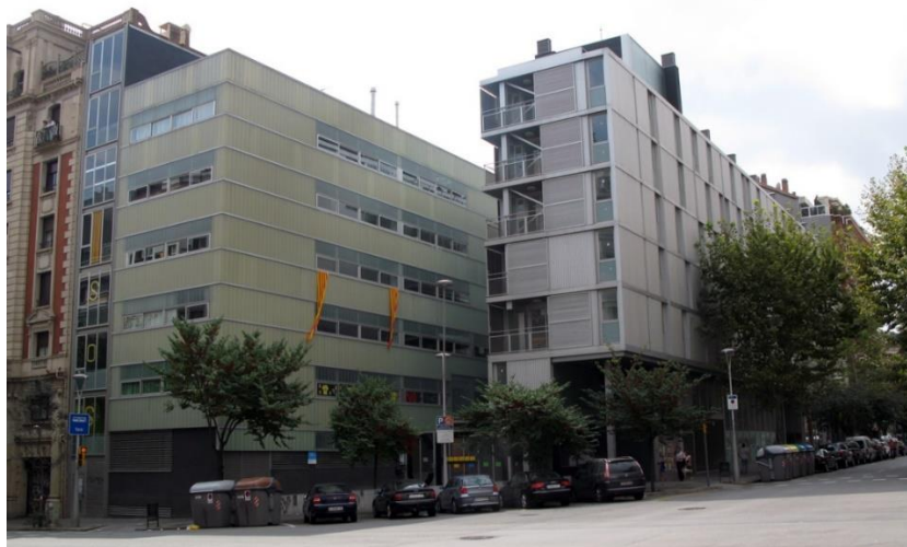
Figure 3. Hybrid complex with housing, school and kindergarden (by J.Coll, J. Leclerc) built in 2001 at c/ Londres in Barcelona
