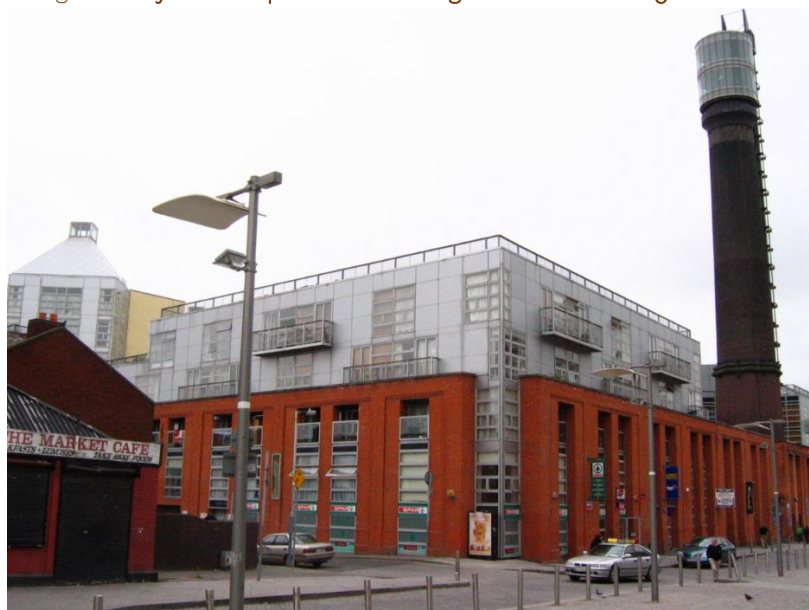
Figure 4. Hybrid complex with housing – Smithfield Village in Dublin
