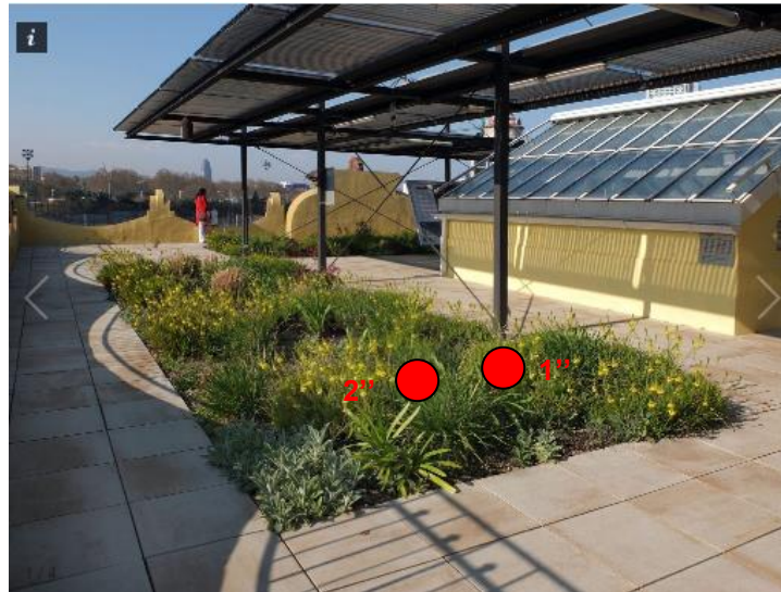
Figure 6. Blue roof in La Fábrica del Sol
