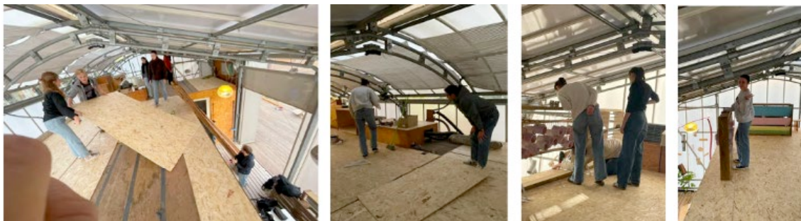
Fig. 7 Refurbishment of LOW3 spaces for community use. Source: Masseck, T. (2023)
