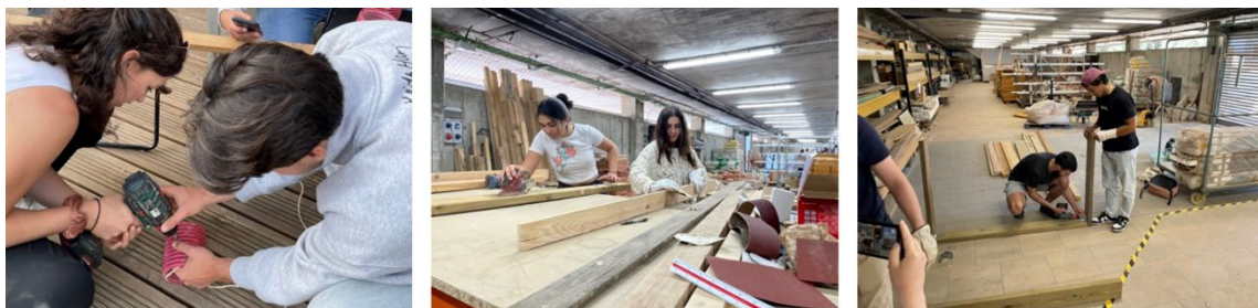
Fig. 5 Construction works of 1:1 scale waste-based shading devices. Source: Masseck, T. (2023)
