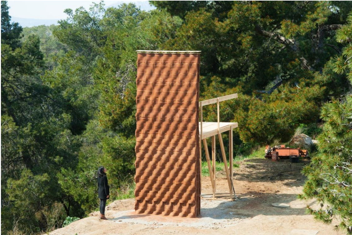
Fig. 3 Digital Adobe final prototype at Valldaura Labs, Bcn. Source: Iaac OTF, Open Thesis Fabrication (2018)
