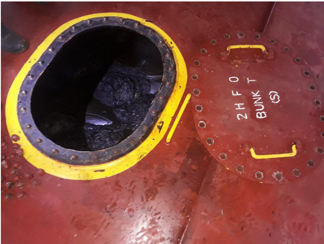
Figure 3. View of VLSFO tank with sludges formation inside. Source: ameydemarine.com
