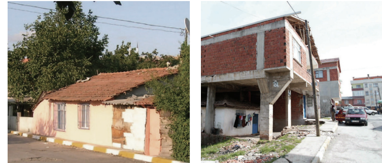
Figures 4, 5. A typical gecekondu and a clear example of residents 'going up,' literally building on top of the original gecekondu to create a new rental market (Balaban, 2011).
