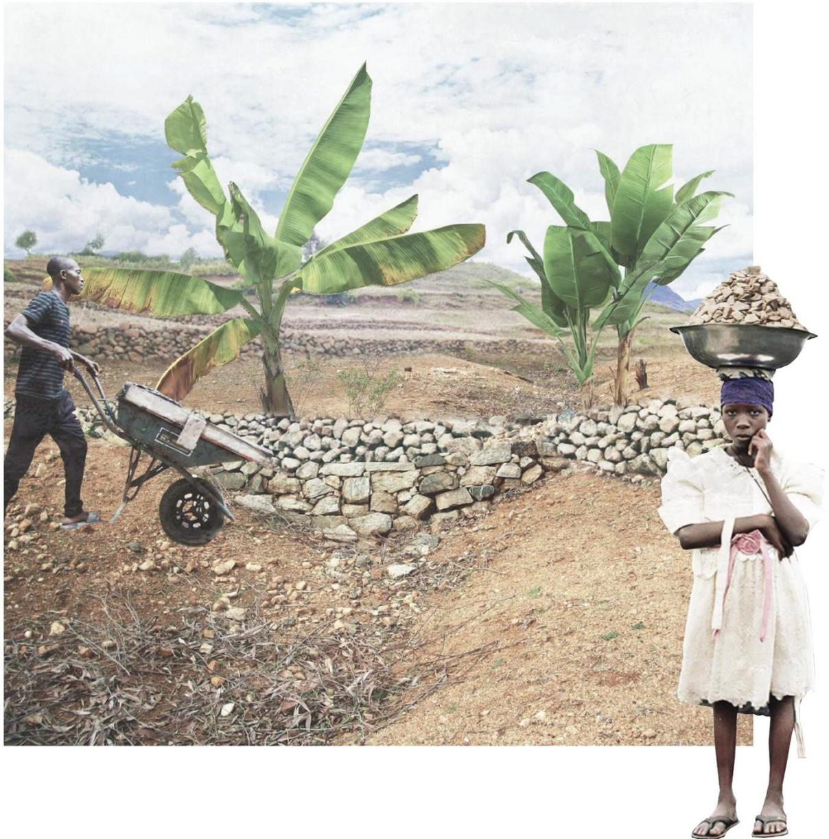
Fig. 12 The recuperation of the landscape starts with a wheelbarrow. The stones are cleaned up from the fields and stacked to form infiltration dams. Banana plants can already be planted since they consume little water. Source:(Van Praet, 2018, pp. 130,131)
