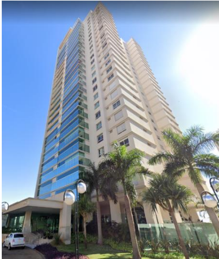
Annex. 2: Pic. 2 – Le Blanc. Source: Google Maps (2022), modified by the authors.
