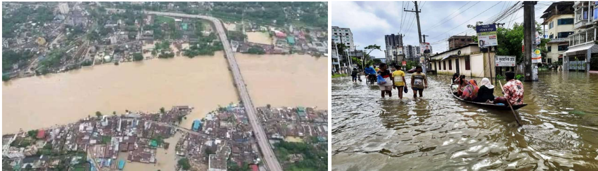
Figure 1. Sylhet city (one of the case study cities) inundated by the worst flood in 2022
