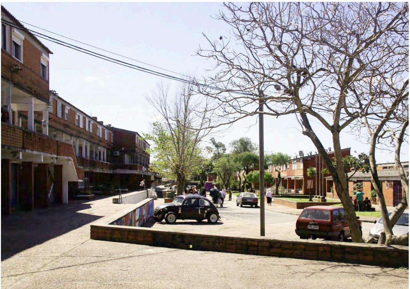
Fig. 01 Mesa 1 Cooperative Housing complex, built from 1971 to 1975, comprises 420 units and several communal facilities. Source: (S.M.A., F.A.D.U. 1981).
