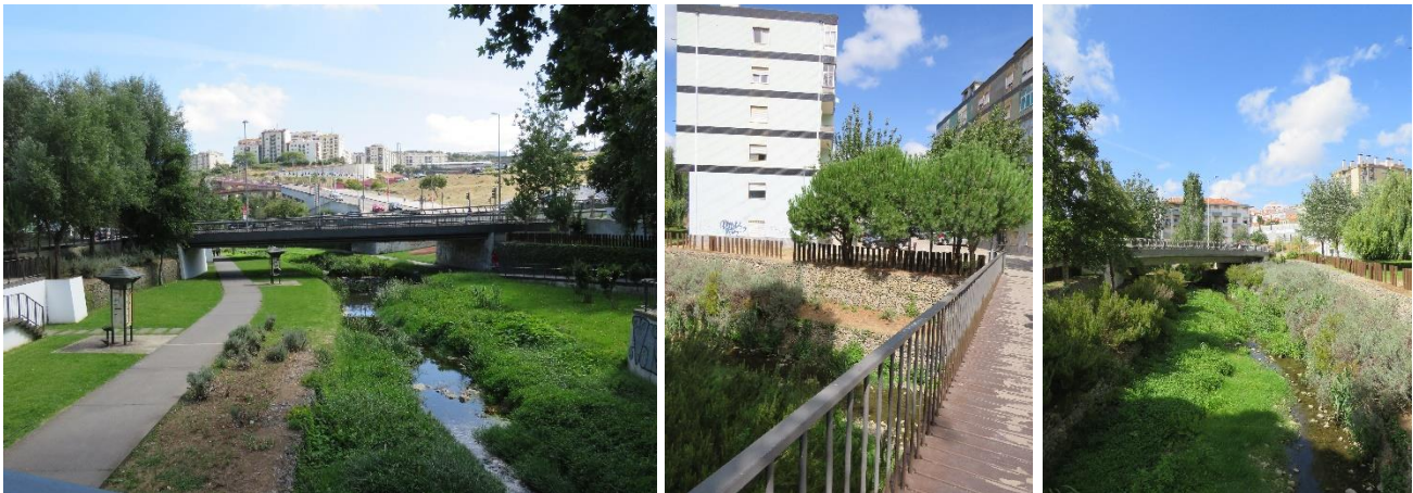
Fig. 07 Polis Cacém operation: Linear Park alongside the Jardas stream
